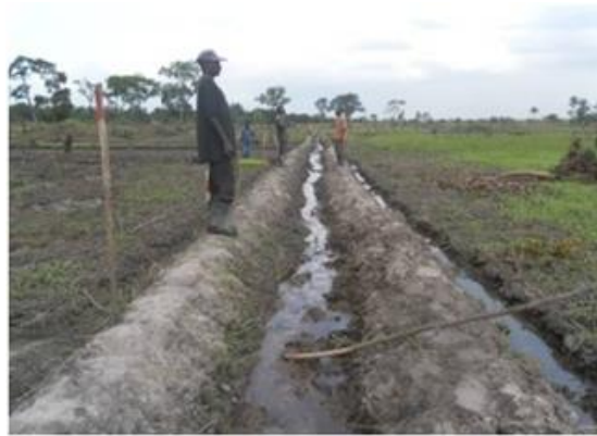
Completed drainage canal [2]
