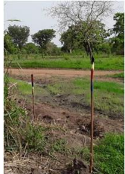
Marking of a belt bund and a point of singularity [3]
